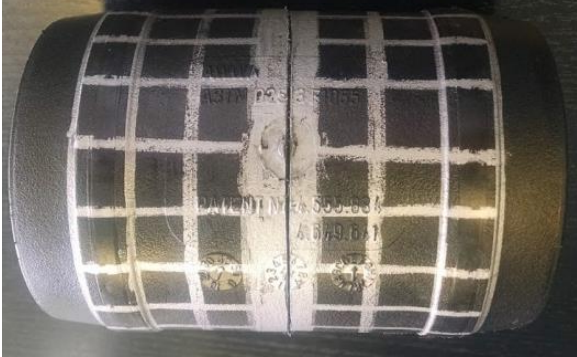
Figure 2: NDT grid on the outside surface of a 2" coupling
